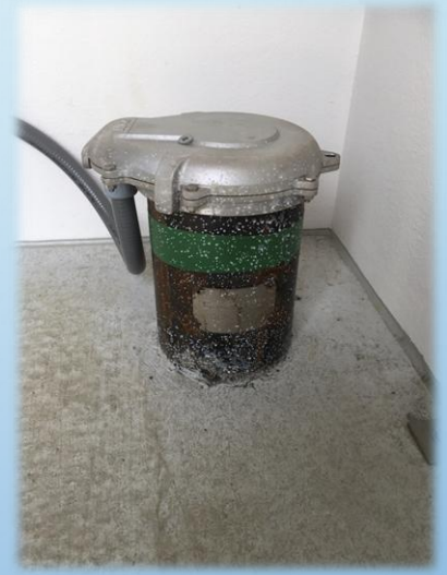
Eel Ground One of two new wells!
