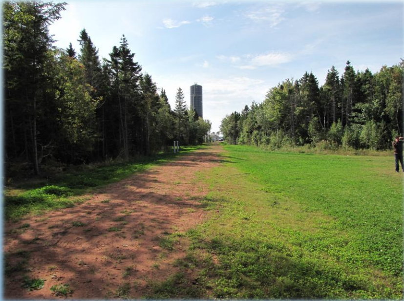
Lennox Is, PEI - well field protected with restricted land use
