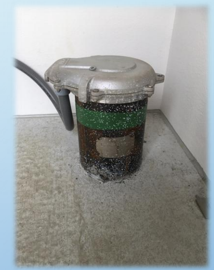
Eel Ground One of two new wells!
