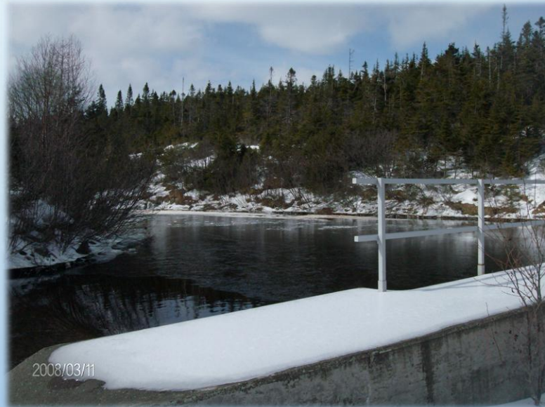
Conne River, NFLD - source water impoundment and screening first step in the treatment process.
